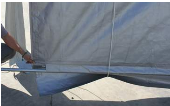
Step 1: Insert the door dropping tube (part #32) into Pocket along Bottom edge of Roll Up Door.
